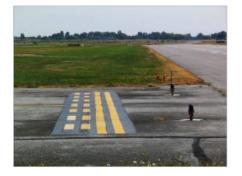
Hold markings Helipad C and B from incursion from vehicles, pedestrian or aircraft. These markings are similar to those near the runways. As with all hold markings, ATC must be contacted prior to proceeding onto these surfaces.
