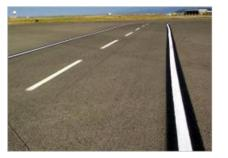
Vehicle Corridors are the roadways for vehicles and equipment operating on aprons, they allow vehicle and equipment movements to occur in a safe and predictable manner.
